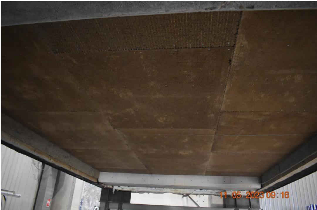
Photo No. 8 Clay boards mounted to the timbre frame.
