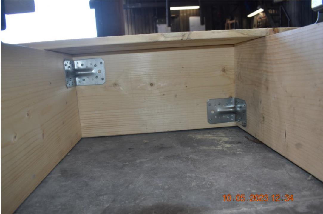
Photo No. 5 Timber joist connection.
