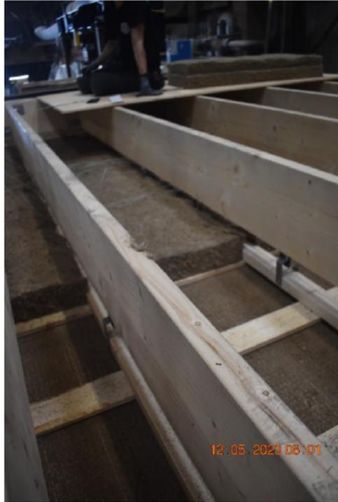
Photo No. 11 Insulation during installation
