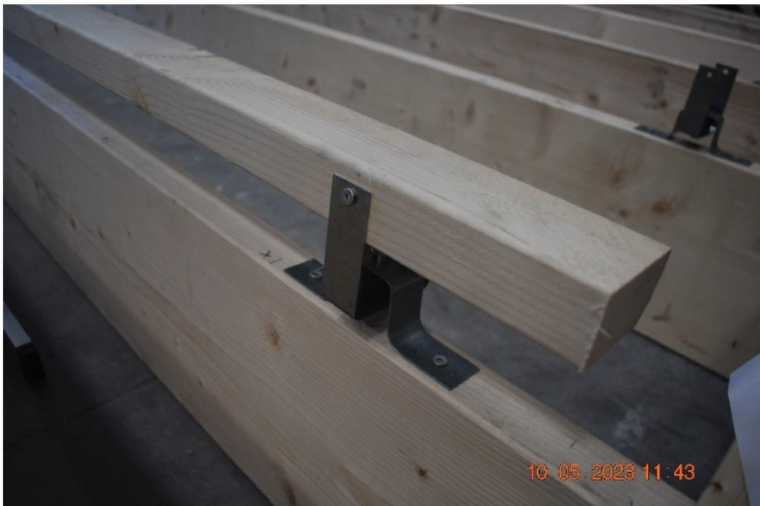
Photo No. 3 Sounds bar installed on the timbre joist.
