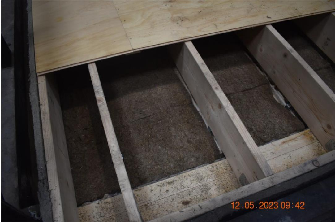
Photo No. 13 Plywood as top layer
