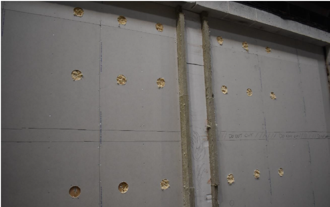
Photo No. 11 Mounting holes for wood fibre insulation.
