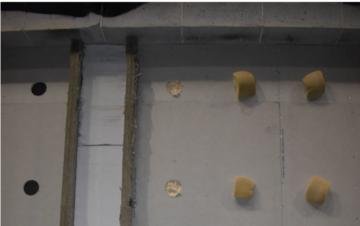
Photo No. 10 Woodfibre insulation.
