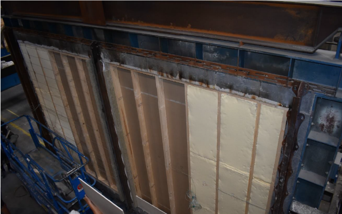
Photo No. 7 Side without wire, insulation slab installed.
