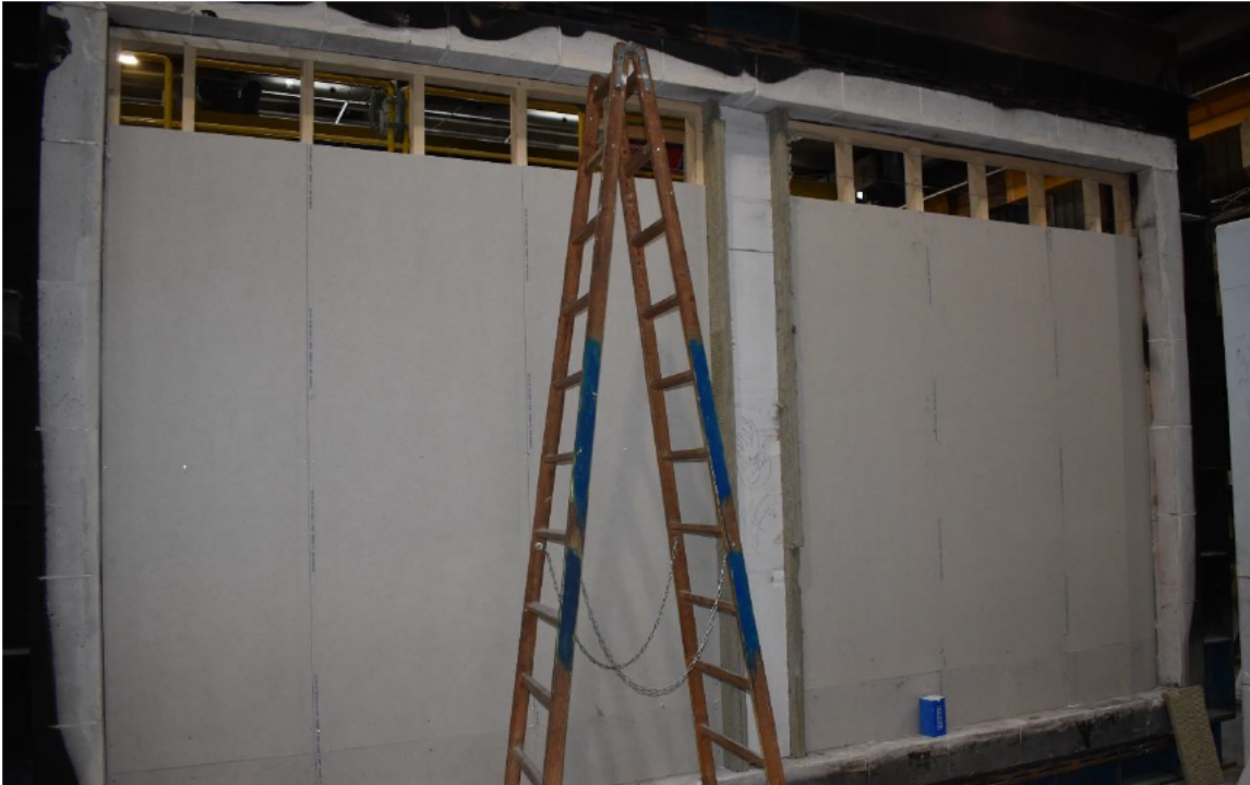
Photo No. 5 Gypsum cladding mounted to studs.
