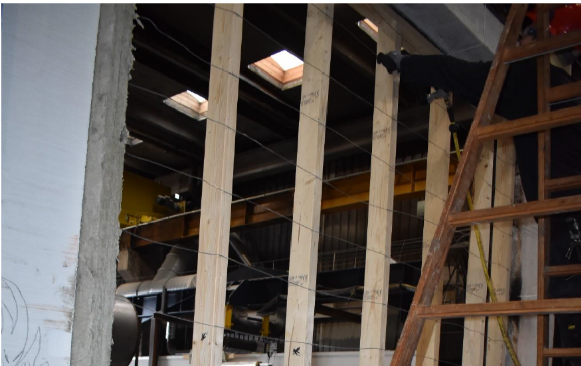
Photo No. 2 Mounting of wiring on timber studs.
