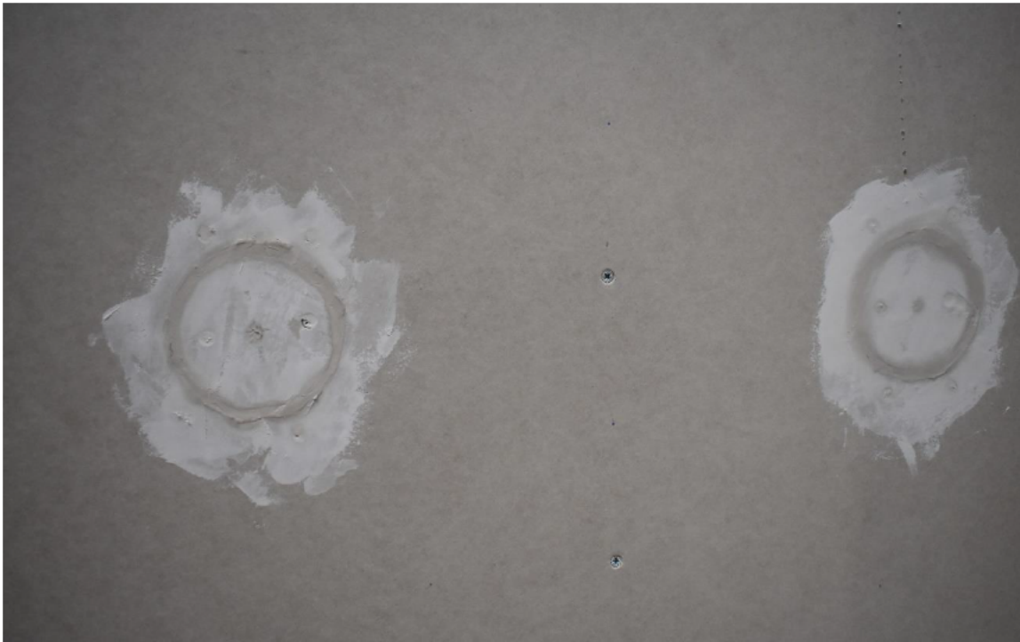
Photo No. 15 Sealed with gypsum mortar.
