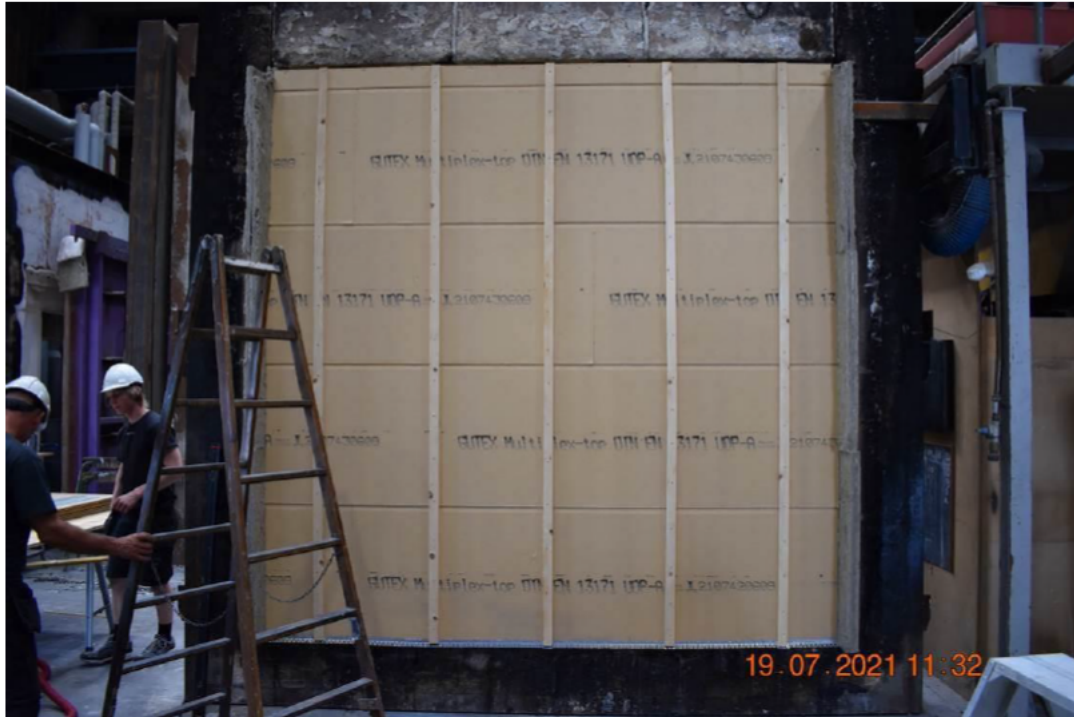
Photo No. 7 Spacer studs is being mounted on the exposed side.
