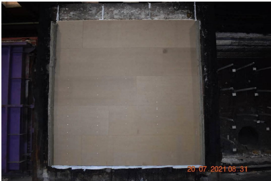
Photo No. 8 Layer of chipboard mounted to studs/spacers on the exposed side.
