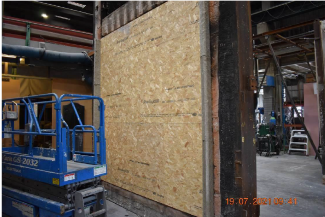
Photo No. 3 Layer of OSB-3 mounted to the studs of the wall on the unexposed side.
