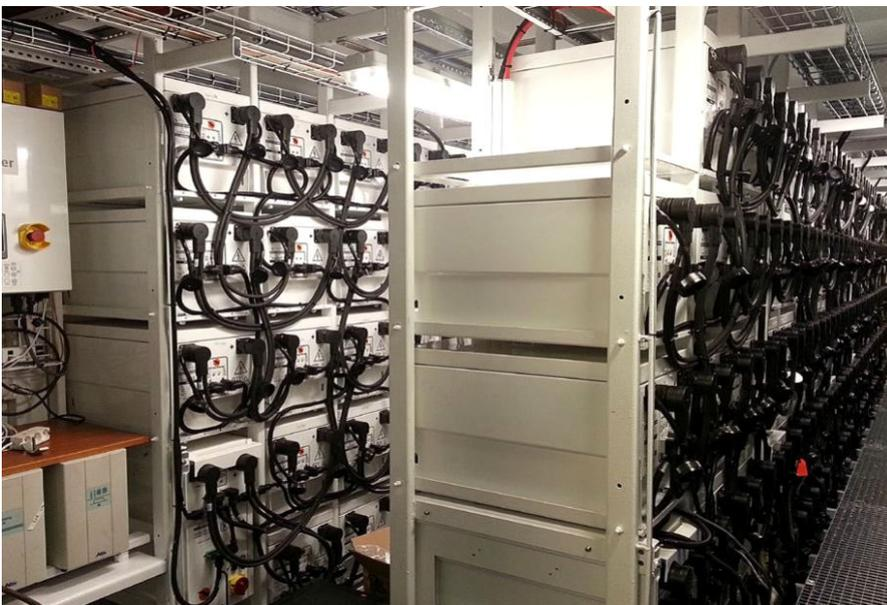
Figure 6: The 1.04MWh battery system on board MF Ampere, Norway. (Source: Corvus Energy)
